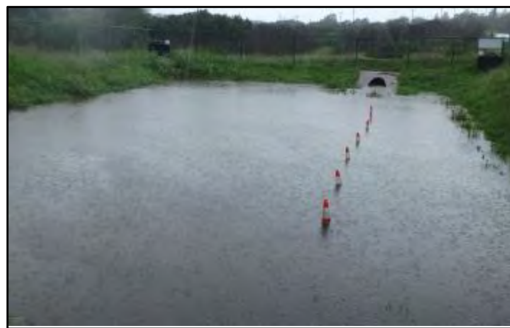
Detention pond holding roadway runoff
